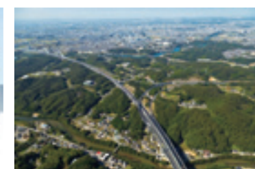
The Shin-Tomei Expressway
