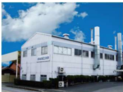
Hekinan Headquarters Factory
